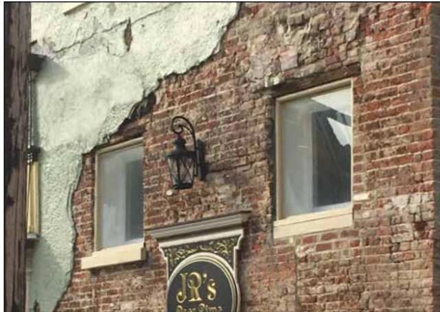
This wall was once stuccoed over, and has not been repointed, leaving a scarred and poorly maintained building in the heart of downtown Smyrna DE.
