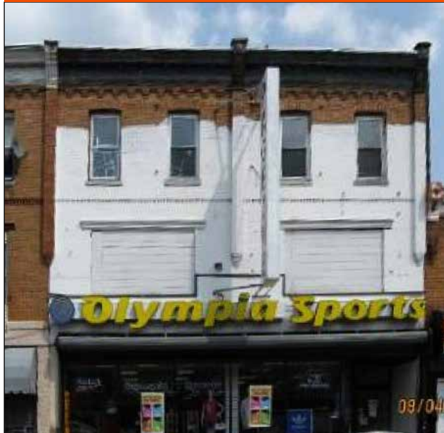
It is not recommended to paint brick (see above), stone, tile, stucco, or molded concrete block if they have never been painted before, as seen on this building in Philadelphia. The unpainted elements have a natural or man-made finish that is important to preserve.
