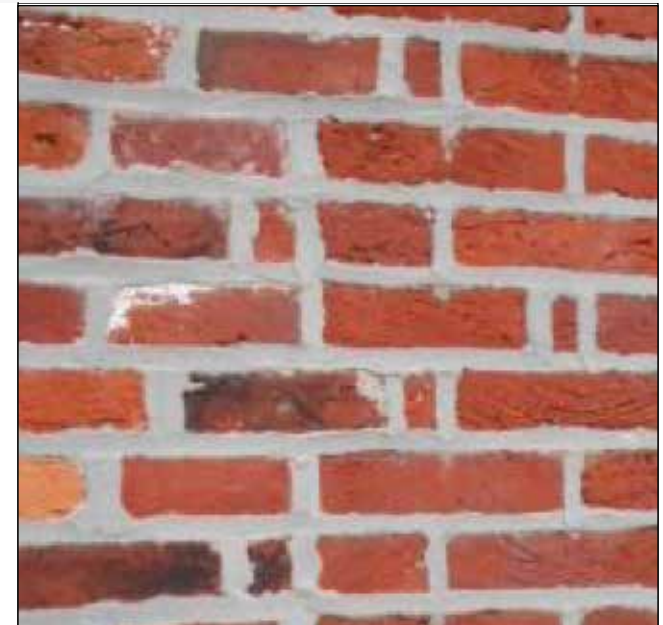
The surface of the brick seen here on a Philadelphia building has been eroded by sandblasting in the past. Sandblasting is not recommended for any masonry or brick building in Seaford.
