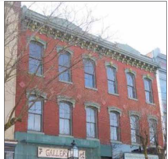
The two over two light replacement wood upper story windows for this building in Bridgeton New Jersey fill the entire window opening.
